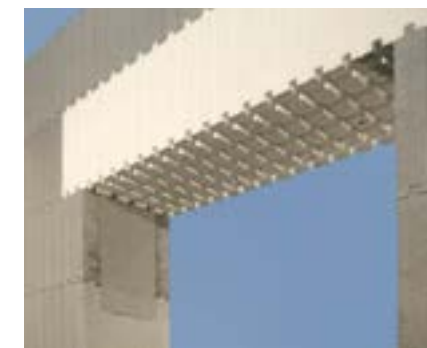
The header element has a U-shaped cross-section.
