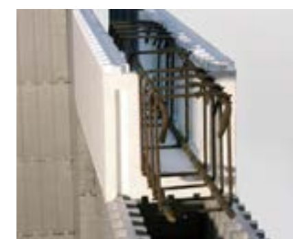
Placement of reinforcement in the ML header element is simple.
