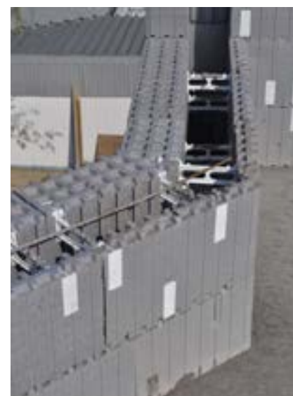
The use of hinge elements to shape corners at any angle.
