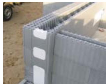
While constructing reveals and blunt wall endings, close up openings in the formwork with OH, OB and OC elements.
